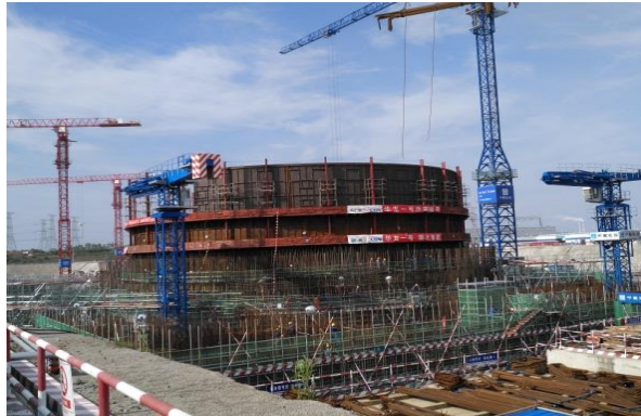
#1NI CW : started in December 2015, Dome Lifting scheduled within the first half of the year 2018
